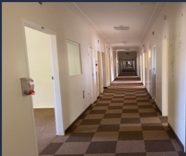
Current condition of former hospital ward
