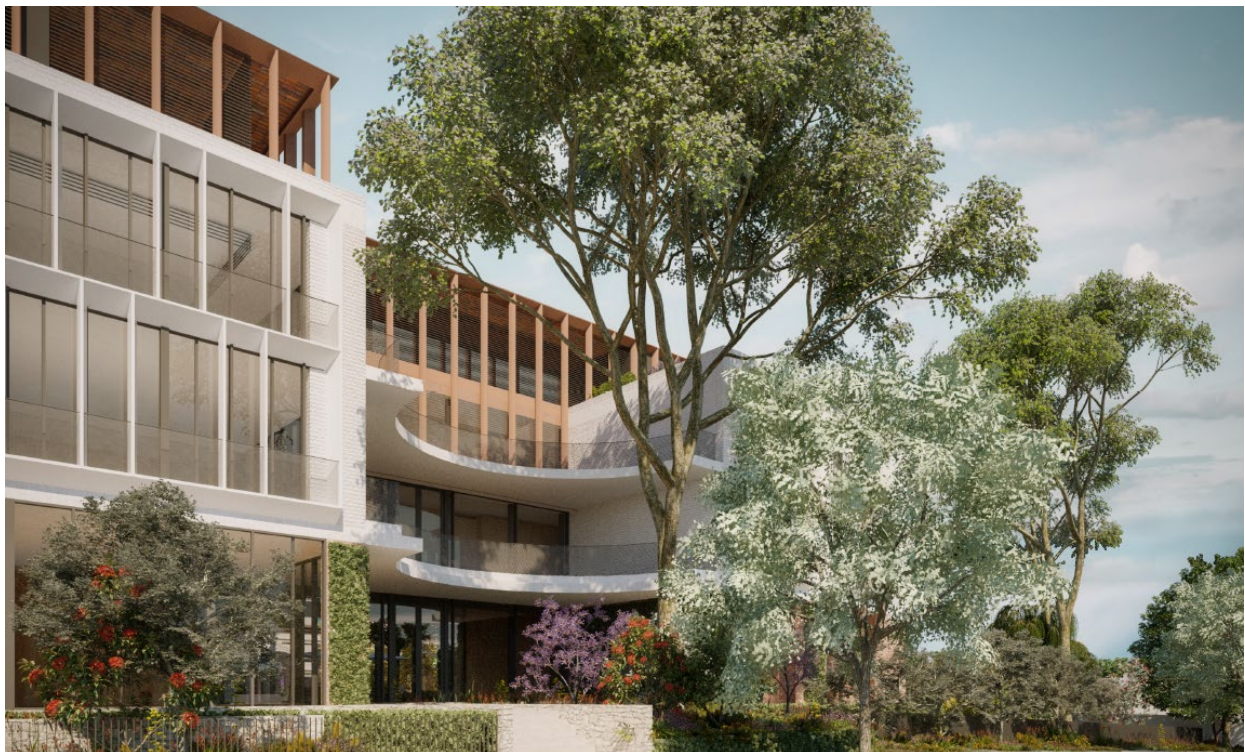
Pedestrian access from Fortescue Street.
